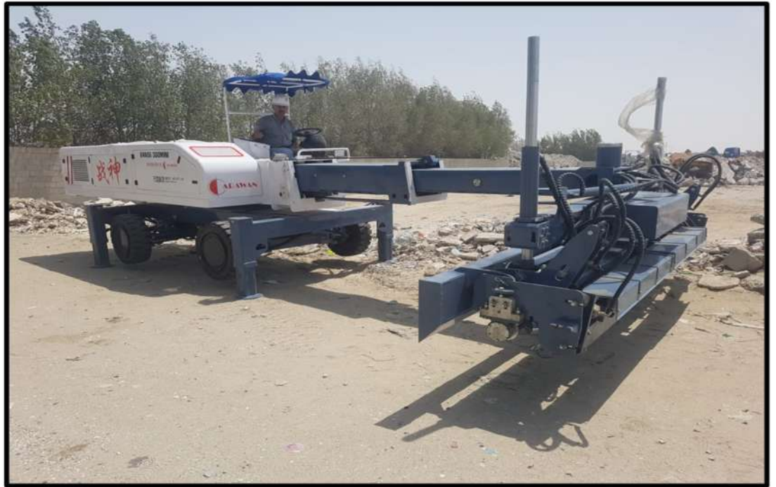
CONCRETE LASER MACHINE VANCE YZ30 - 4
